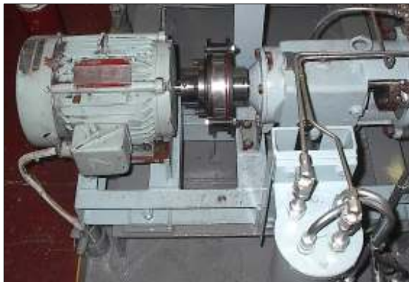
MGE-07, 20HP, 3600RPM, Oil & Gas, Oil Transfer Pump, Oil Tanker
