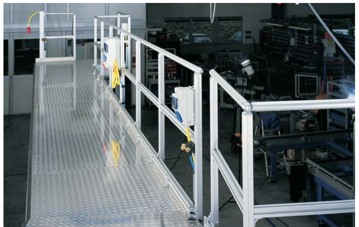
Guardrail posts built from mk profile technology can be used to attach various components, e.g. electronics supply equipment
