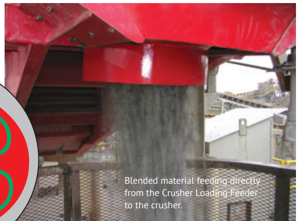
4-inch rock being distributed through the peripheral discharge of the Crusher Loading Feeder.
